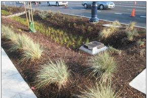
Figure 3-7. Example Infiltration Basin Figure 3-8. Exam Source: Montana Post-Construction Storm Water BMP Design Guidance Manual
