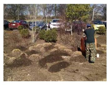
Figure 17. Mulch replacement is one activity that may be included in a maintenance agreement for stormwater practices such as bioretention.
