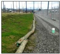
Figure 3-4. Example of Proper Construction BMP Source: HDR, Inc.
