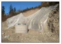
Figure 3-5. Example of Poor Construction BMP
