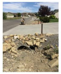
Figure 3. Roadside Ditch and Culvert Mapped in Residential Area
