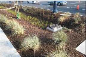
Figure 3-6. Example Infiltration Basin Figure 3-7. Exam Source: Montana Post-Construction Storm Water BMP Design Guidance Manual
