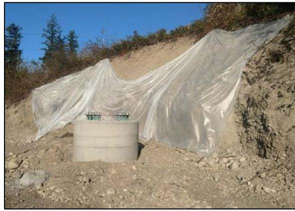
Figure 3-2. Example of Poor Construction BMP
