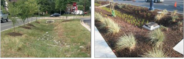
Figure 3-4. Example Infiltration BasinFigure 3-5. Example Bioretention AreaSource: Montana Post-Construction Storm Water BMP Design Guidance Manual
