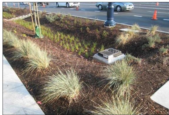
Figure 3-5. Example Bioretention Area
