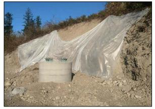
Figure 3-2. Example of Poor Construction BMP
