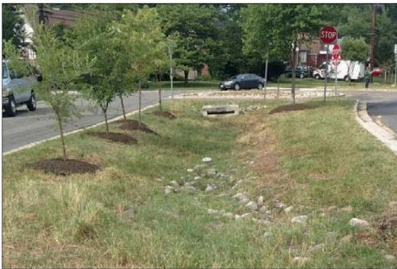
Figure 3-4. Example Infiltration Basin
