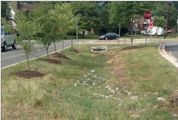
Figure 3-7. Example Infiltration Basin
