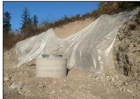
Figure 3-5. Example of Poor Construction BMP
