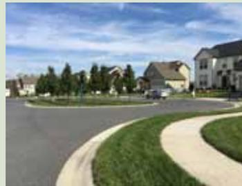
2. This loop lane reduces the need for backing up of vehicles and creates about 10% less impervious cover than Option 1.
