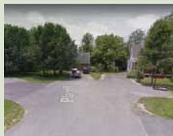
4. This hammerhead or t-shaped turnaround produces about 80% less impervious cover than Option 1. This alternative is good for very short (< 200 feet) streets. (Photo Source: Google Earth)
