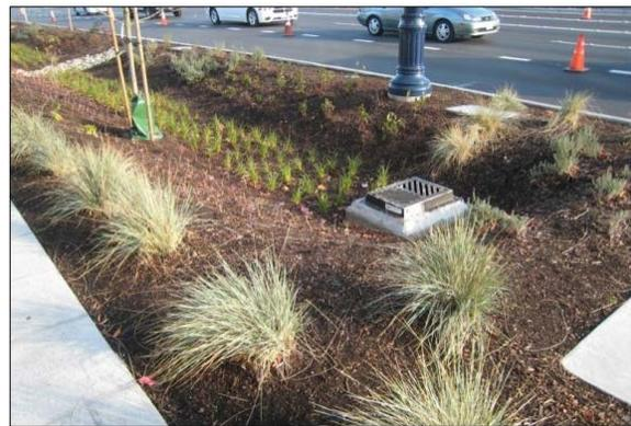
Figure 3-8. Example Bioretention Area
