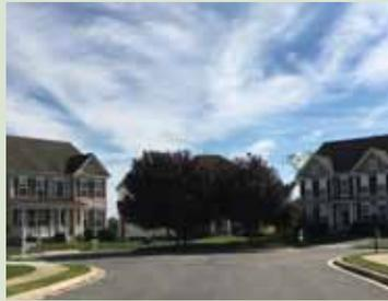
3. This cul-de-sac also has a 50-foot radius but incorporates a vegetated island. This alternative creates about 15% less impervious cover than Option 1.
