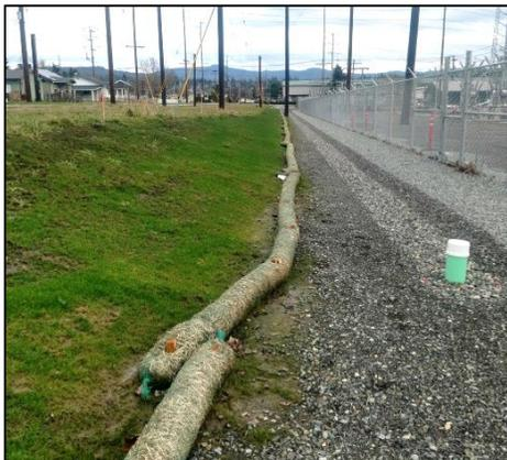
Figure 3-3. Example of Proper Construction BMP
