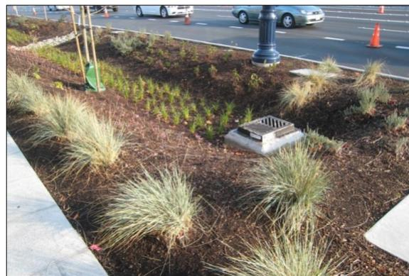
Figure 3-7. Example Bioretention Area
