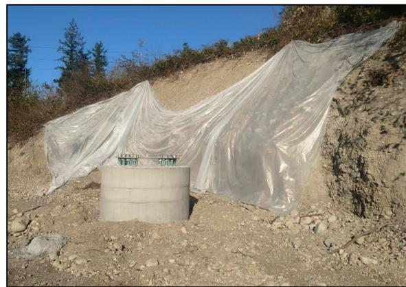
Figure 3-4. Example of Poor Construction BMP
