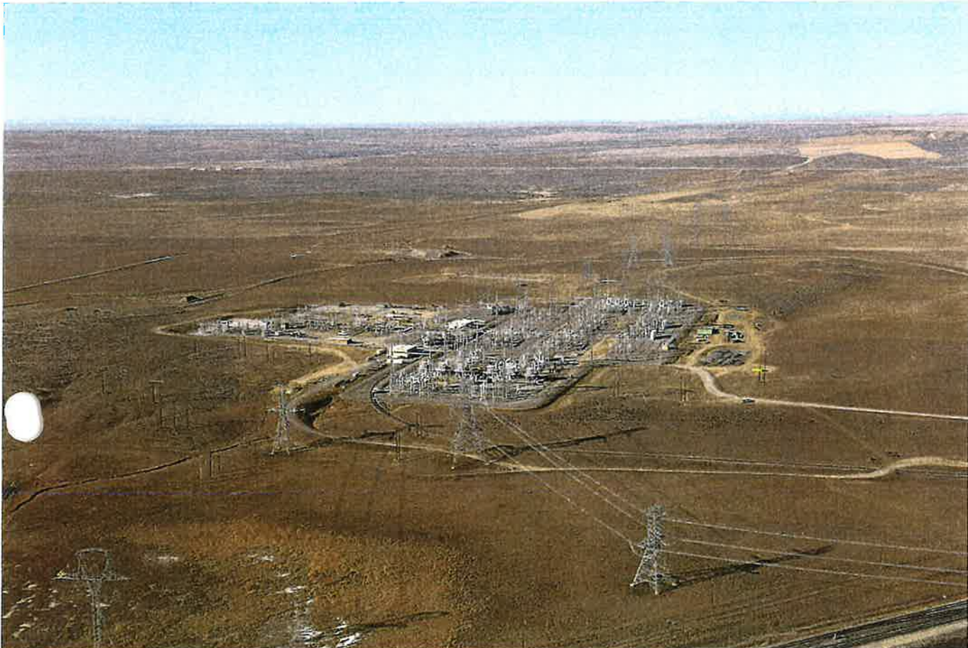
An aerial view of a Quantica Infrastructure substation facility.
