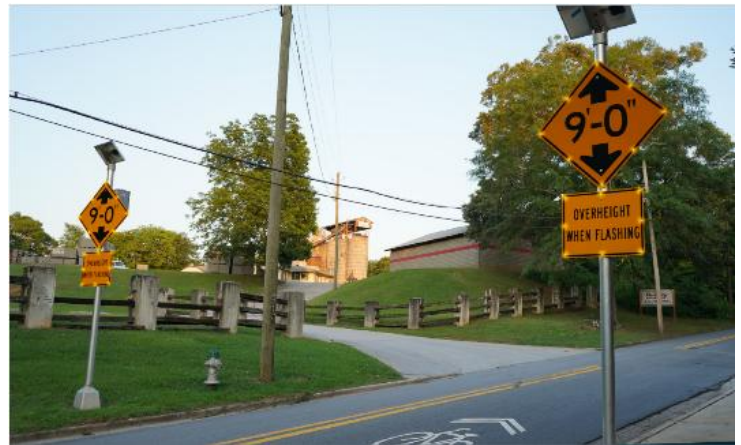
FIGURE 9. EXAMPLE OF A VERTICAL CLEARANCE WARNING SYSTEM
