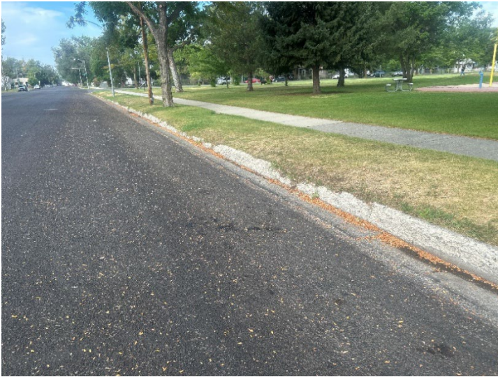
Deteriorated curb and gutter at Highland Park.
