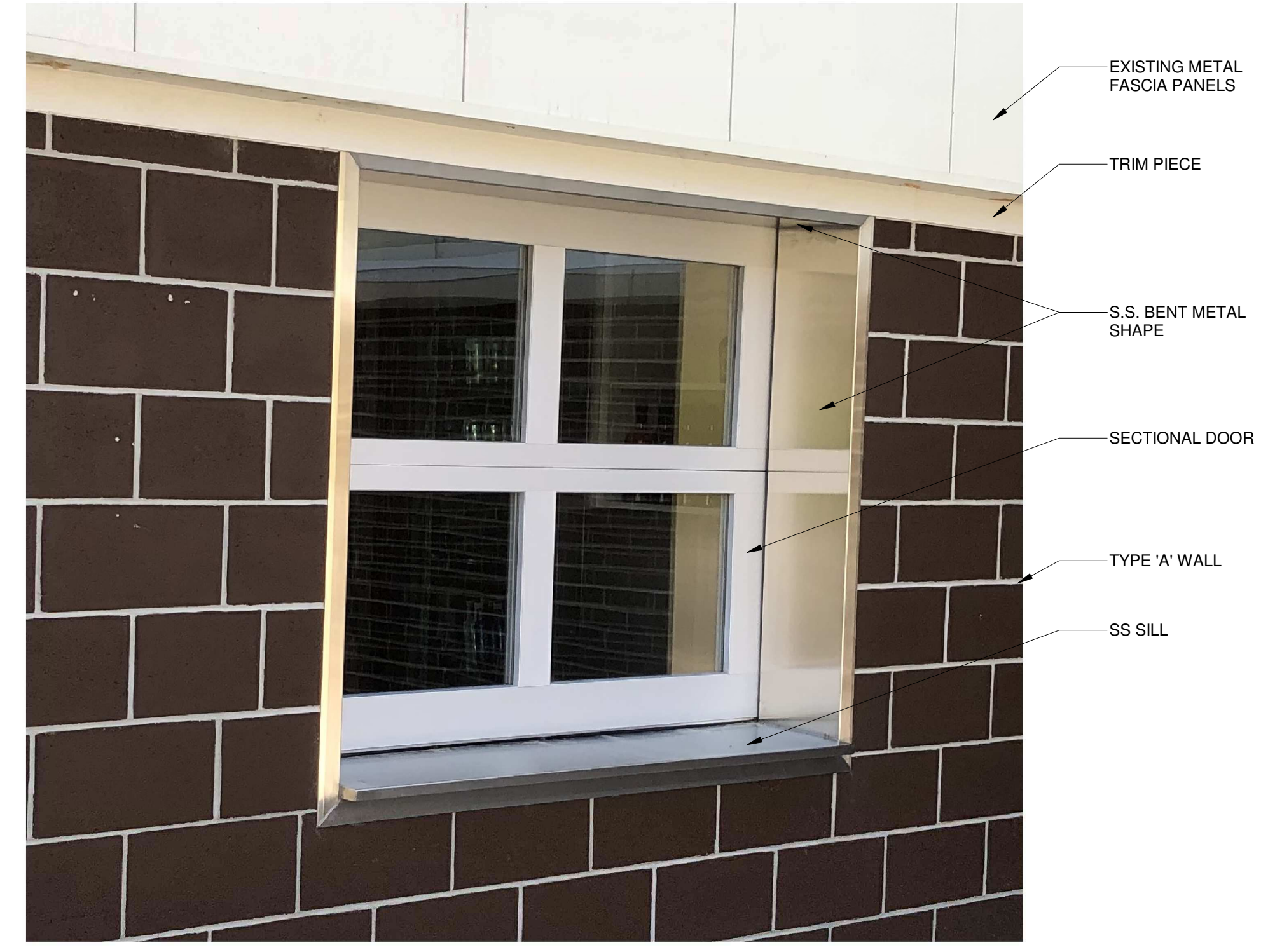
EXTERIOR WINDOW AT EXISTING CONCESSION
