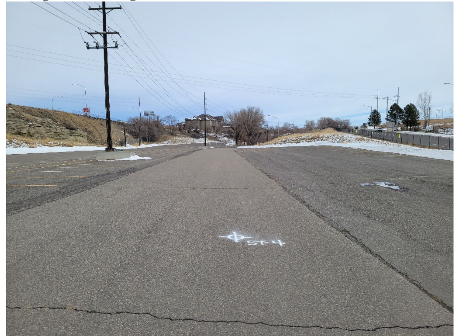
Boring ST-4, looking east.
